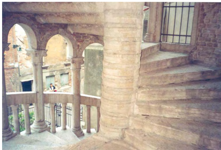
Figure 102. Venice, Bovolo Staircase. Illustrating the wide steps and broad newel and demonstrating how highly visibility user of the stair would be. Photographer: C. Ryder.
