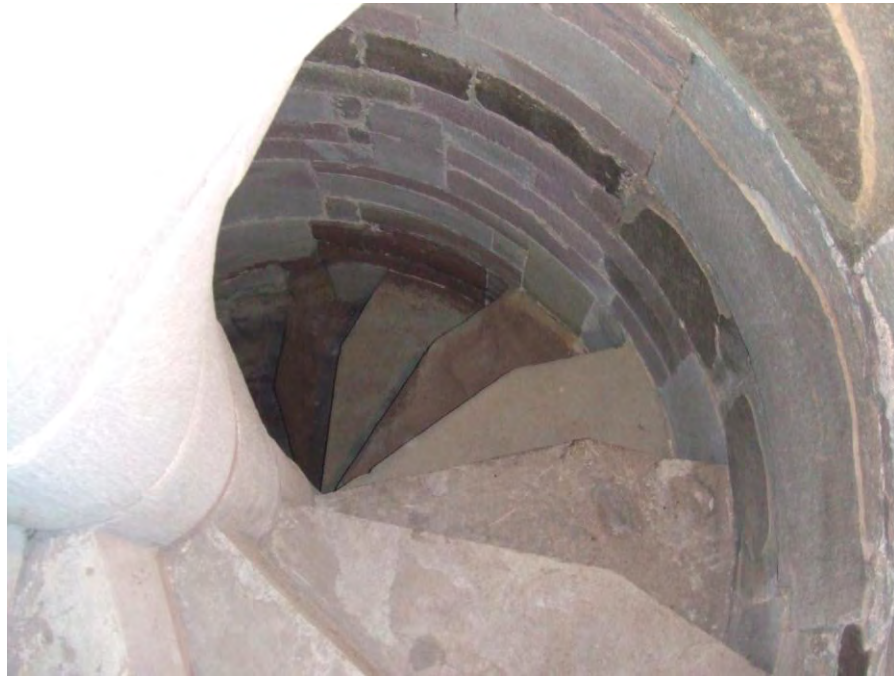
Figure 6. Wenlock Priory: Prior's House Spiral. Illustrating how the edge of the step is cut away to facilitate movement on the double spiral stair. Photographer: C. Ryder.
