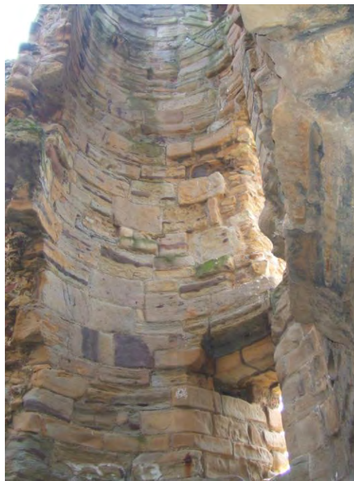
Figure 68. Flint Castle North-West Tower. Illustrating spiral stair shaft. Photographer: C. Ryder.
