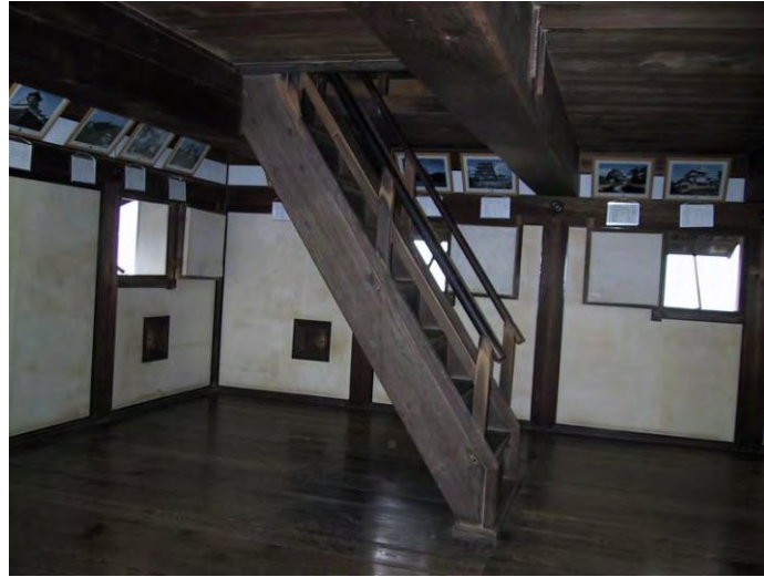
Figure 12. Kochi Castle: Interior Stair. Illustrating typical tenshu interior stairs. Photographer: E. Obershaw.
