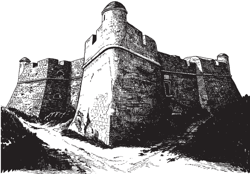
Fort du Montalban, Nice, 1559–61. Fort Montalban, situated on top of Mount Boron, dominating the city of Nice on the French Riviera, was built between 1559 and 1561 by the Italian engineer Domenico Ponsello. Fort Montalban was intended to control and defend the passage between Nice and Villefranche-sur-Mer. It was a massive square with four bastions placed at the angles.
