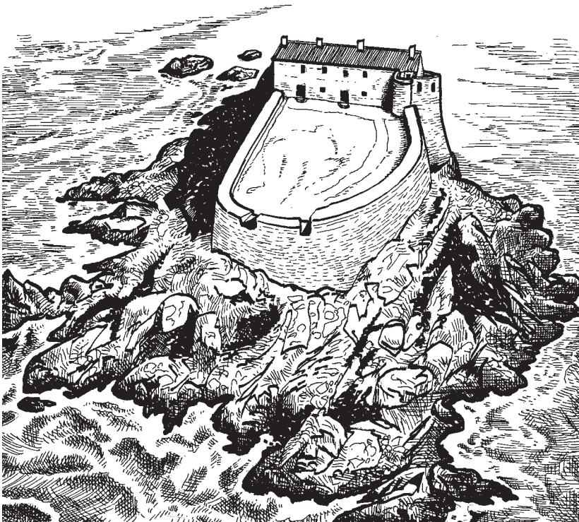
Fort de la Conchée (Saint-Malo). La Conchée Fort, designed by Vauban in 1693 and completed in 1695, is built on the small, rocky island Quincé, four km. northwest of Saint-Malo. Its plan completely deviates from classical bastioned principles. The fort consists of a service building placed on high and thick masonry walls, forming a wide oval gun battery with embrasures turned towards the open sea. The fort was declared obsolete in 1889. Today, it is a nature reserve for seabirds.
